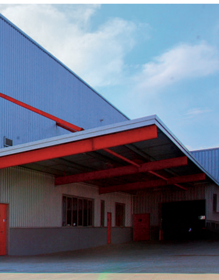
EJOT Fastening Systems in Taicang, China
