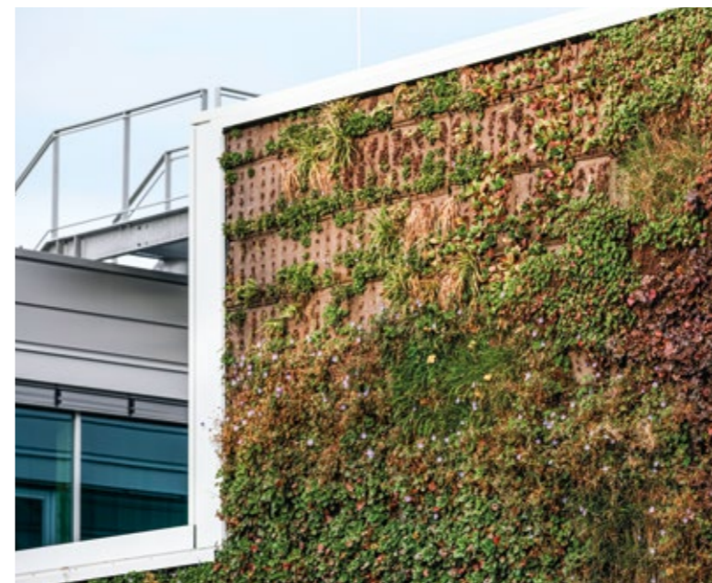
Green facade on the west side of the TEC CENTER.
